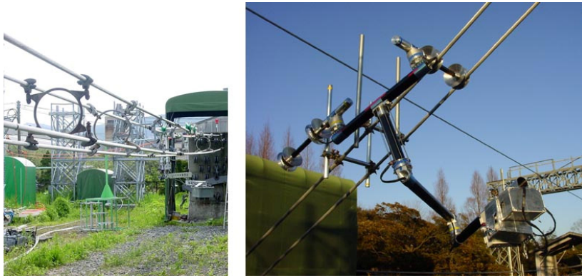
Fig. 9 – Cable spacers (left) and Expliner crossing obstacle on inclined cable (right).
