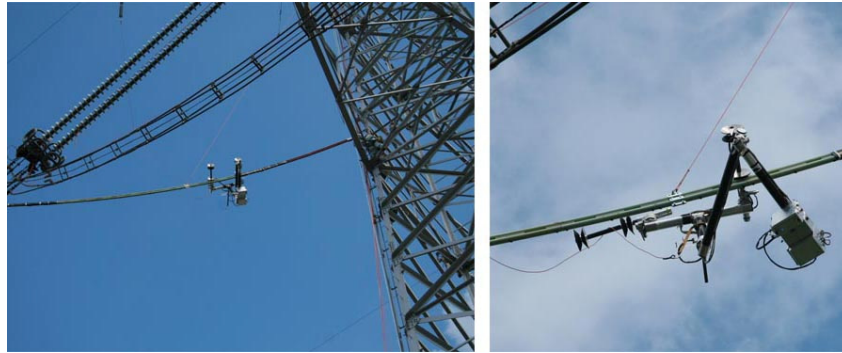
Fig. 11 – Expliner moving on loading pipe (left) and performing an automated motion.
