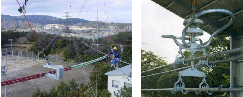
Fig. 2 – Loading pipe between tower and cables (left) and clamp suspender (right).
